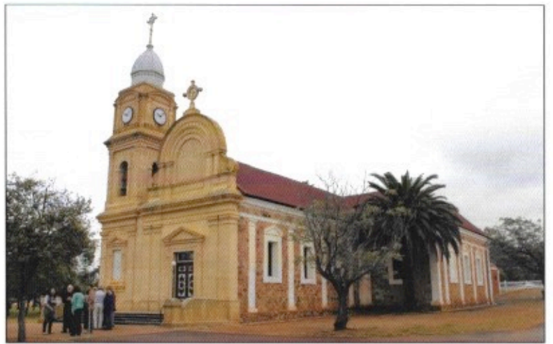
The Abbey Church at New Norcia, north of Perth. Society member and Benedictine resident of New Norcia, Father Anscar, hosted a tour of the church and other facilities at the monastic town, for those attending the Clan Society's Gathering in Perth
