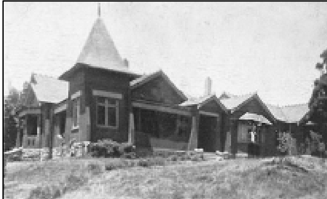
The larger house at Qambah in 1951
